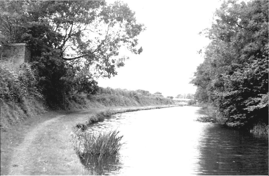
PLATE 3. The Lancaster Canal at Garstang looking north in 2001. The bridge seen from the north in Plate 1 is removed leaving the bridge abutments now overgrown with shrubs and trees. Beech ( Fagus sylvatica ) trees line the canal on the right. Shade from the trees and boat traffic from the nearby Garstang Marina limit the growth of emergent aquatics but the towpath is mostly vegetated. Photo: E. F. Greenwood.
